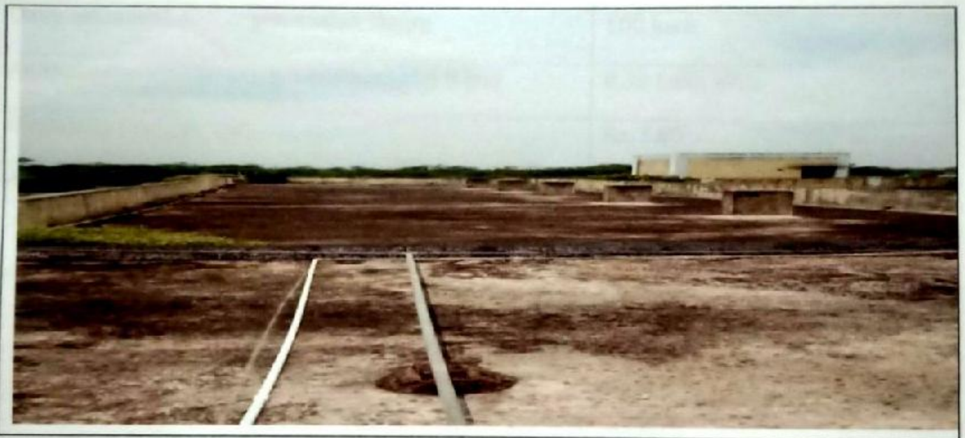
Proposed Site for 10kwp Solar Power Plant
